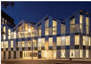
22 Handyside Street is built of lightweight concrete and steel. The steel frame was designed by Arup, which also helped devise a construction methodology working in 7m sections to avoid too much heave on the ground, with the lowest point 800mm from the crown of the tunnels. BAM built 750mm-deep strip foundations with a bespoke lightweight concrete with stringent QA procedures, and Jablite infills.
