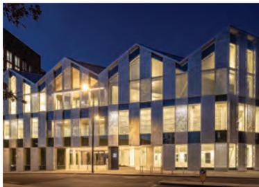
22 Handyside Street is built of lightweight concrete and steel. The steel frame was designed by Arup, which also helped devise a construction methodology working in 7m sections to avoid too much heave on the ground, with the lowest point 800mm from the crown of the tunnels. BAM built 750mm-deep strip foundations with a bespoke lightweight concrete with stringent QA procedures, and Jablite infills.
